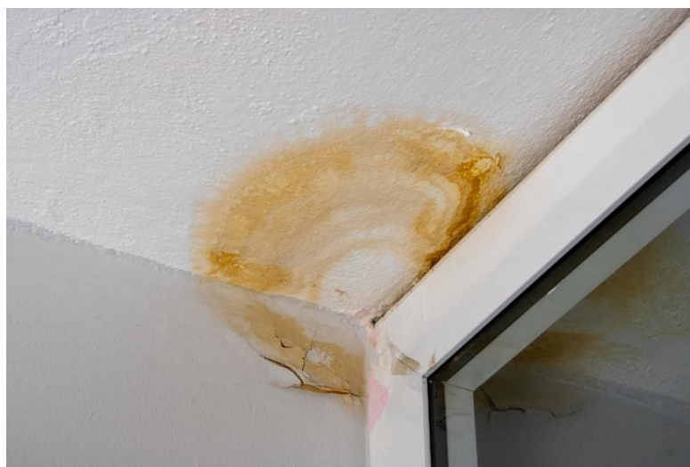
Figure 1: Mould and mildew growth at ceiling [2]
