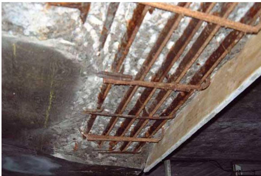
Figure 2: Corrosion of concrete at rebar [2]
