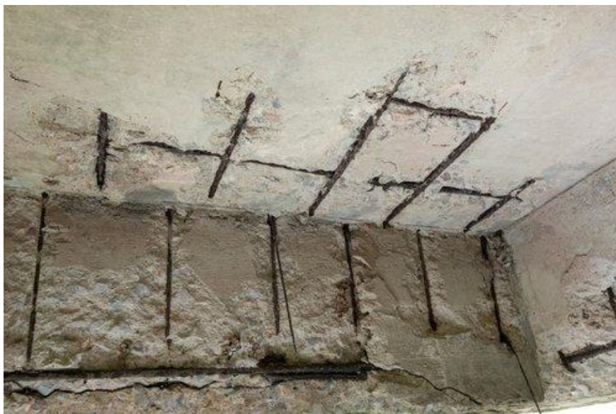
Figure 1: Concrete spalling [1]
