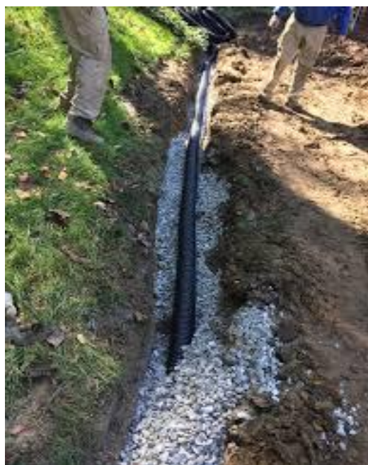
Figure 2: French drain installation [3]
