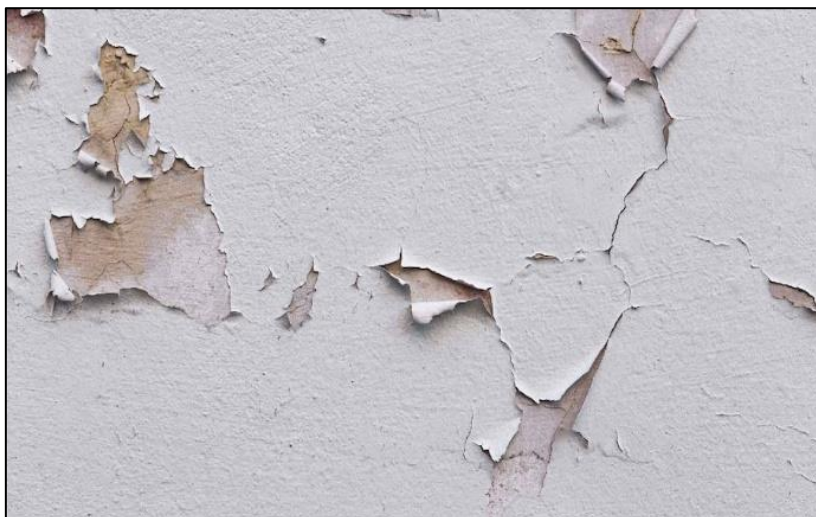
Figure 2: Peeling Paint due to Water Damage [4]
