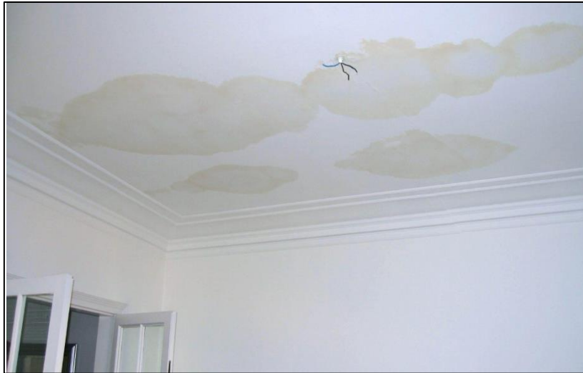
Figure 1: Yellowish Stain at the Ceiling [3]
