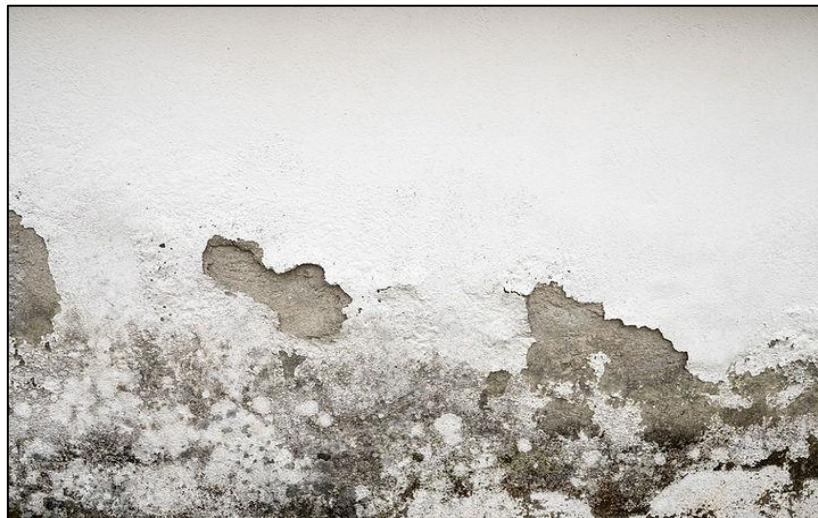
Figure 4: Peeling paint due to water damage [7]
