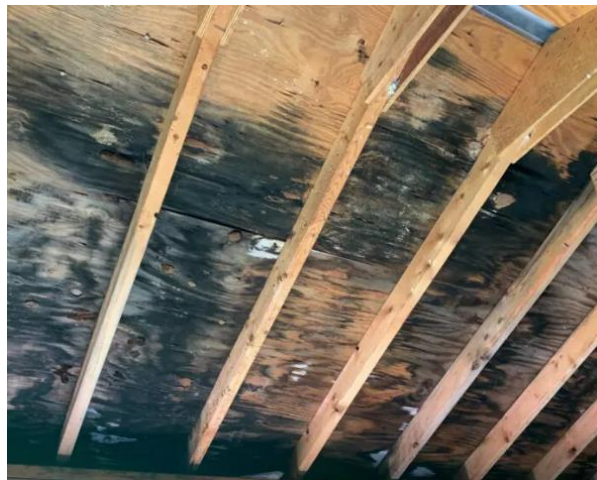
Figure 1: Mould Growth [1]
