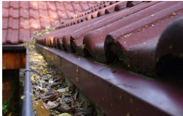
Figure 3: Clogged Gutters [3]
