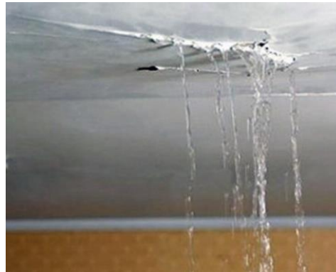
Figure 2: Roof Leaking [2]
