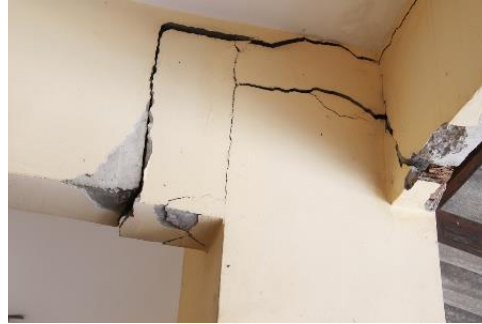
Figure 3: Cracks on the Wall and Floors [6]
