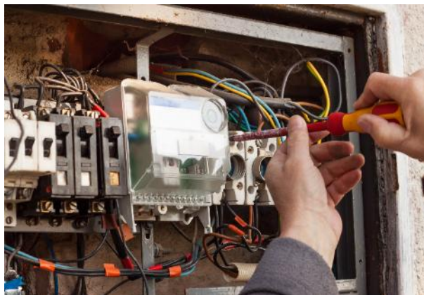
Figure 4: Repairing Distribution Box [9]
