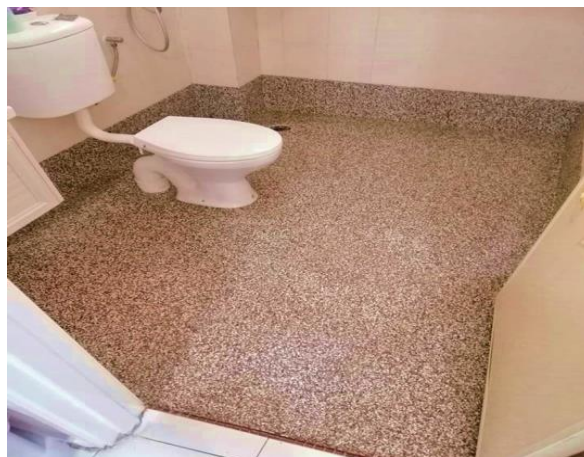
Figure 1: Epoxy Resin Coating in Toilet
