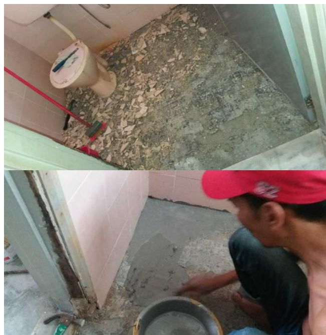
Figure 2: Cementitious Waterproofing in Toilet
