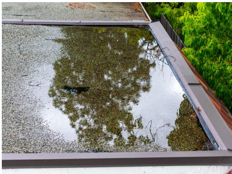
Figure 4: Water Ponding [4]
