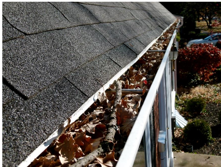
Figure 1: Clogged Gutter [1]
