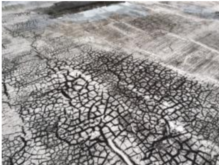
Figure 2: Roof Alligating [2]
