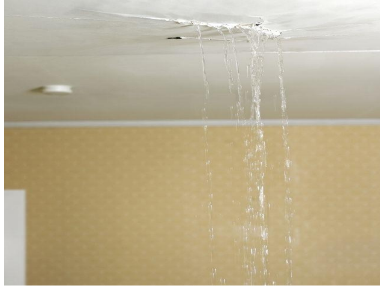
Figure 3: Roof Leakage [3]
