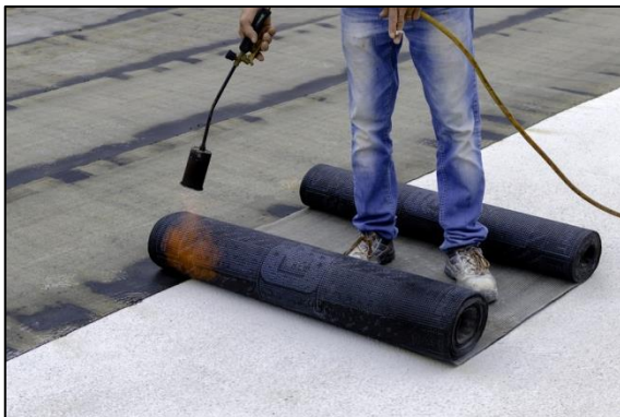
Figure 1: Bituminous Sheet Membrane
